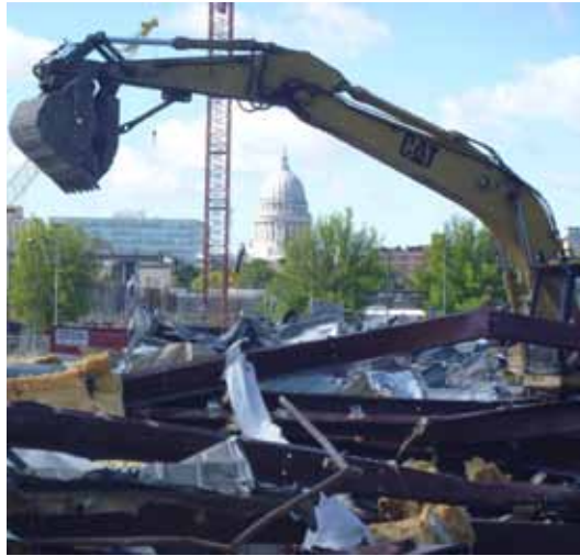
Don Miller site during deconstruction (photo by Bob Shaw)
